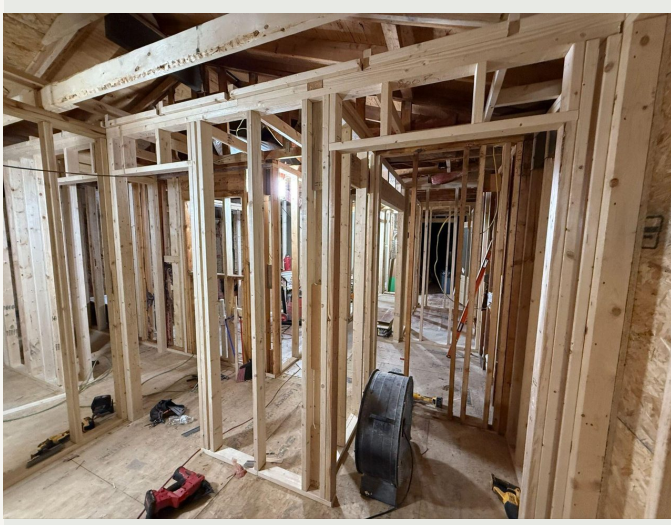
Interior wall framing
