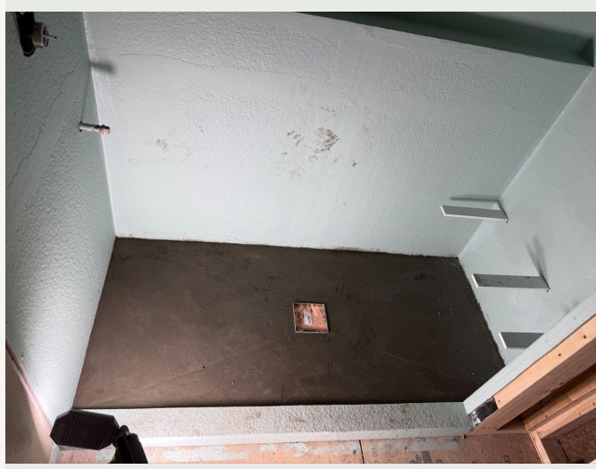
Interior construction progress
