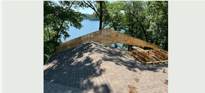
Roof framing progress
