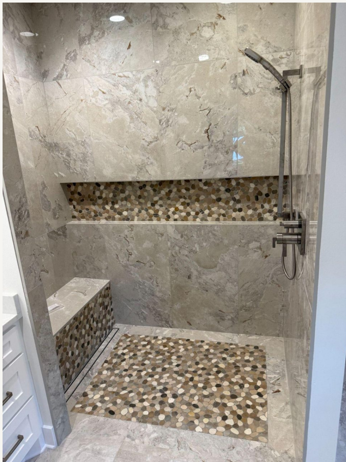
Primary shower: wall and mosaic tile
