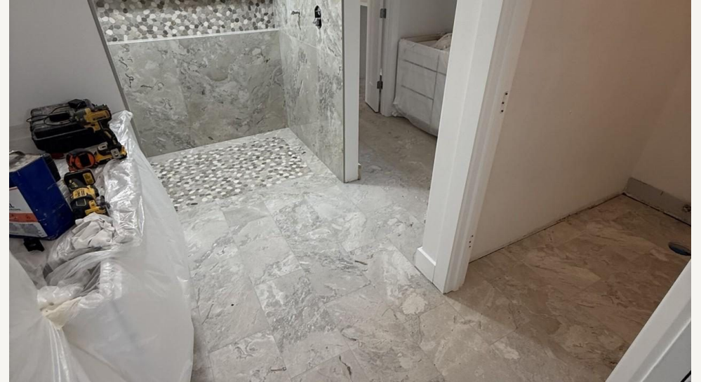
Shower threshold and adjacent floor tile
