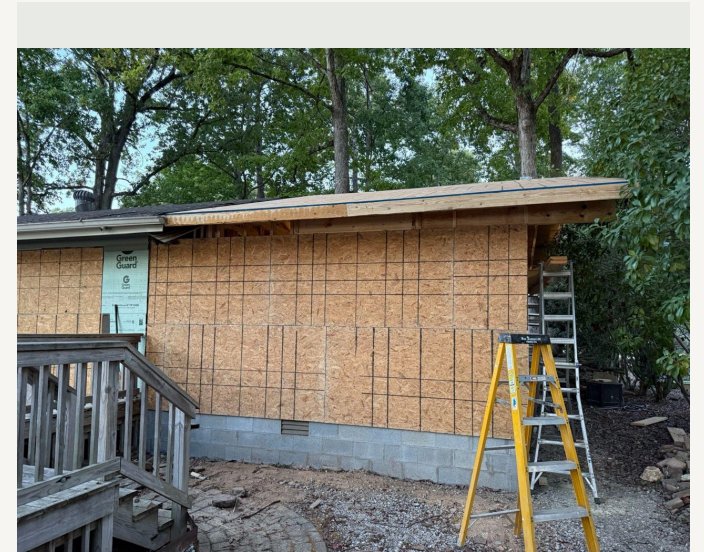
Exterior addition progress
