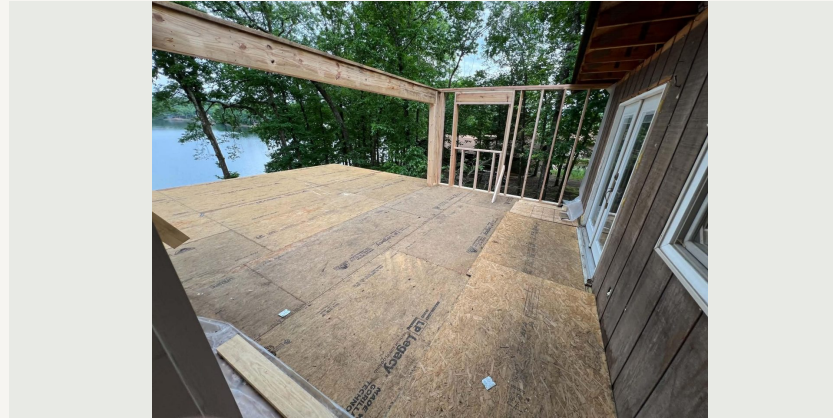
Deck construction progress
