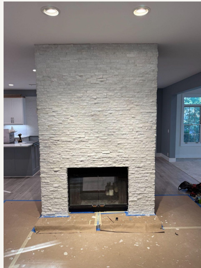
Fireplace: veneer installation
